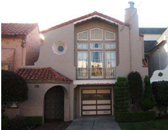
The "Surprise House," 1548 35 th Avenue.
